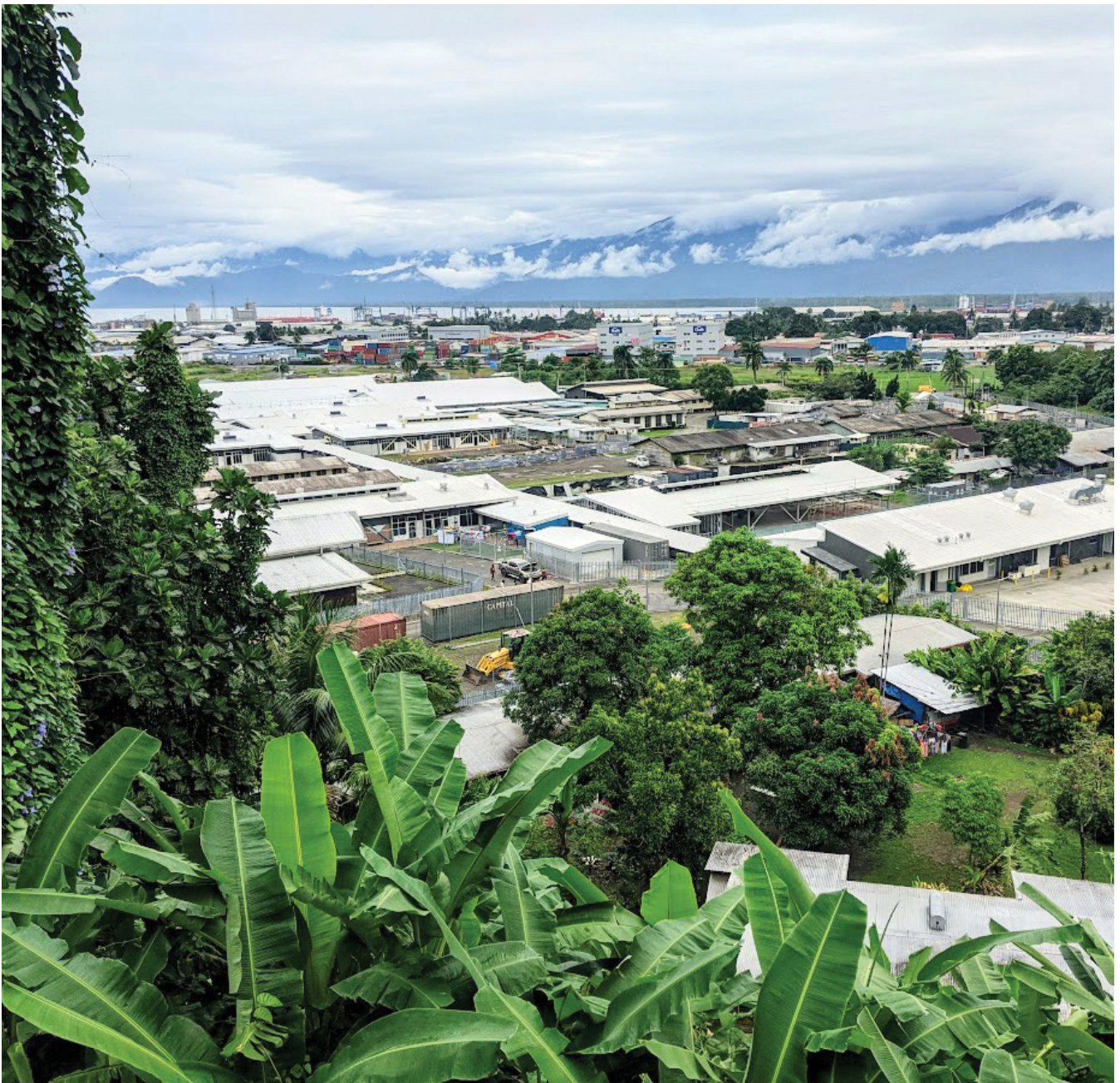
Image below: Construction of the new ANGAU hospital in Lae, Papua New Guinea. Photo by JP Miller.
