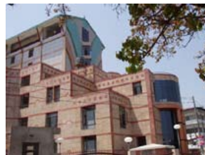
Bir/NAMS Emergency and Trauma Centre under construction
