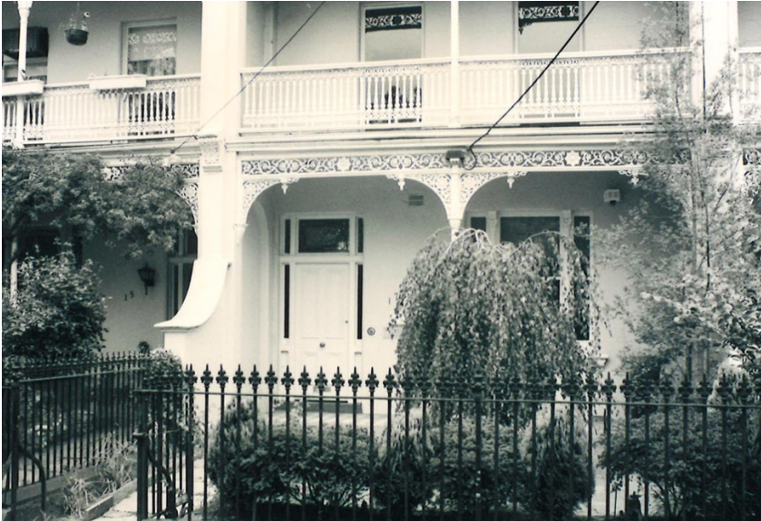
The façade at 17 Grattan St, Melbourne.
