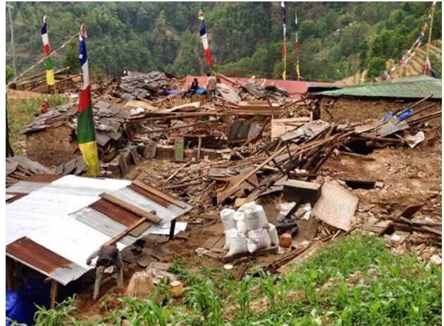
A badly damaged hill village
